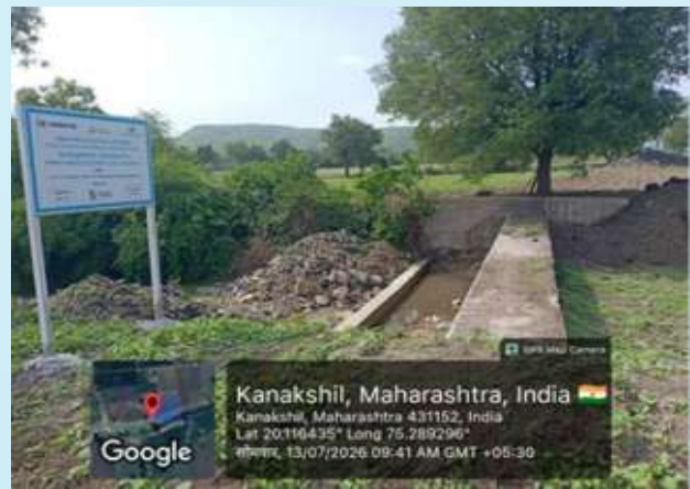
Repair work of existing checkdam structure at Kanakshil village, Khultabad tehsil, Chhatrapati Sambhajnagar
