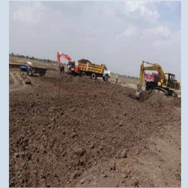
Desilting site at Jalkawadi Reservoir
