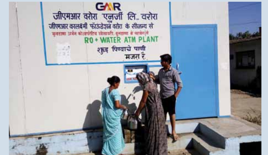
Reverse Osmosis water ATM plant, Majra Rai, Chandrapur District
