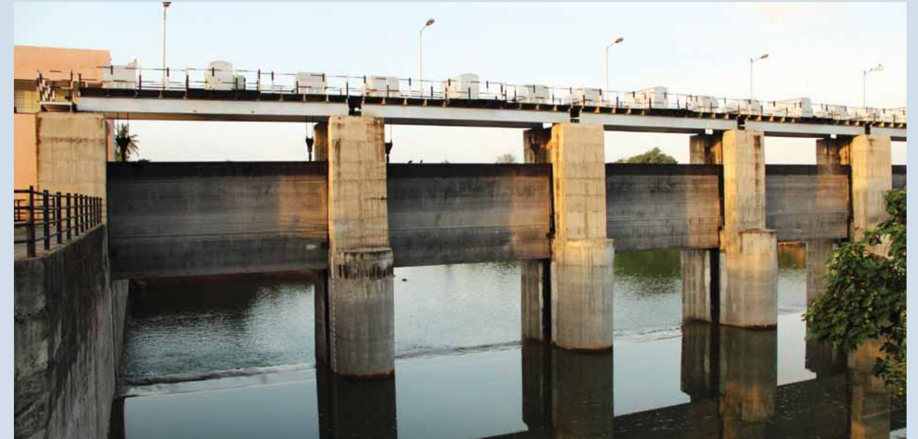
Bhekleswar Dam, Ronaj village, Kodinar Taluk, Gir Somnath District, Gujarat
