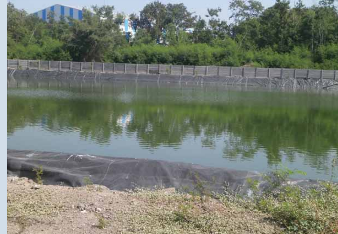
Rainwater harvesting pond
