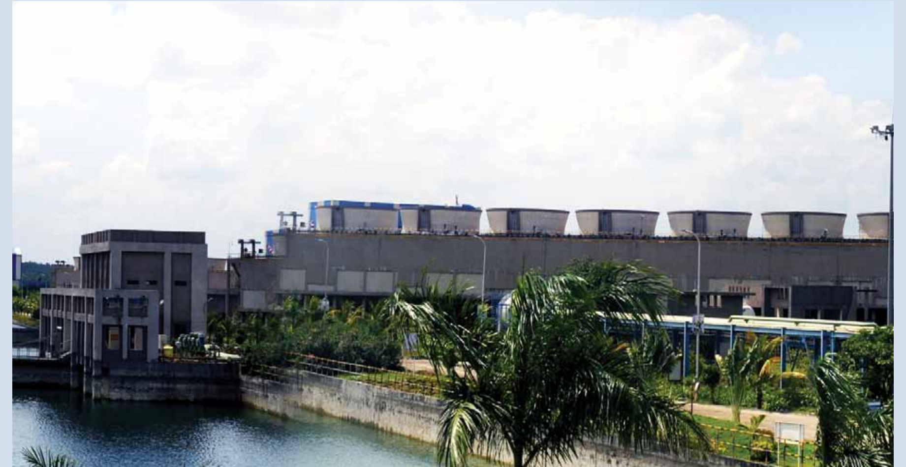
Cooling tower using polymer technology
