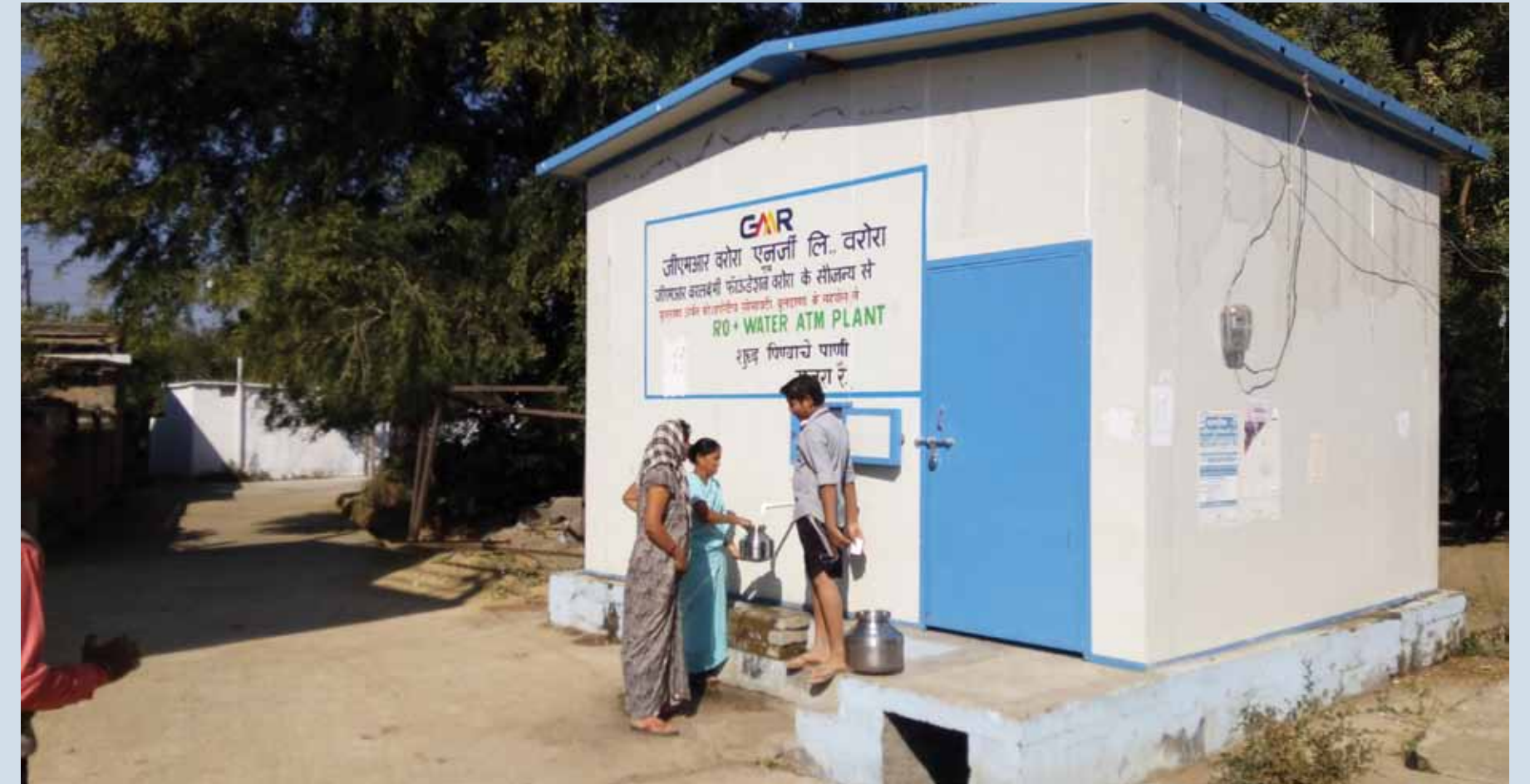
Reverse Osmosis water ATM plant, Majra Rai, Chandrapur District
