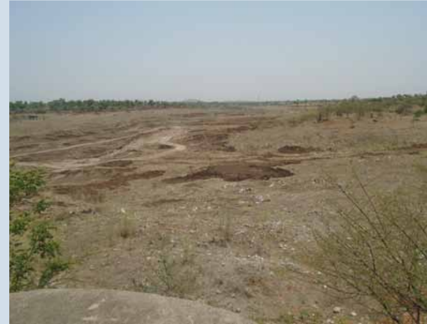
Before: Ganga Sagar dam (Percolation tank) Dhamari Site
