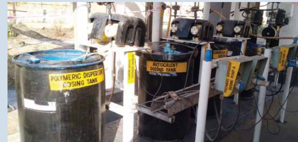
Polymeric dispersant dosing system for polymer technology
