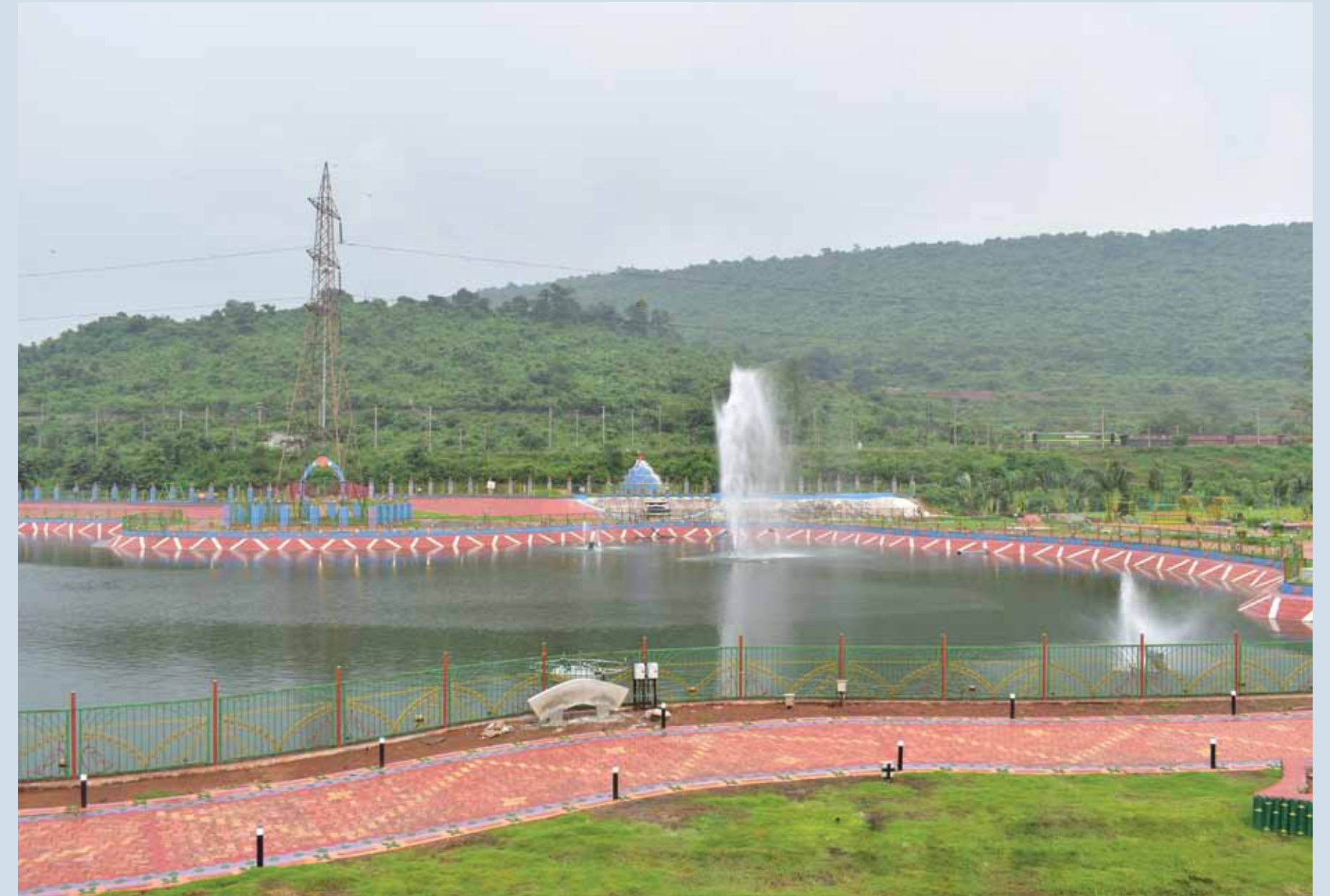
Storage cum percolation tank, Joda, Odisha
