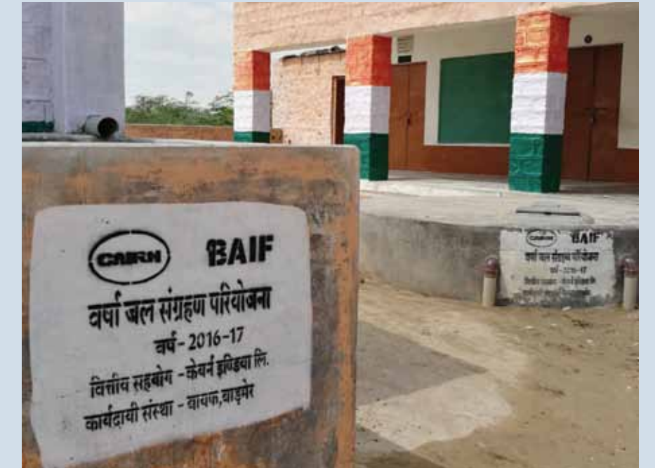
Roof water harvesting structures at Adarsh Dhunda School
