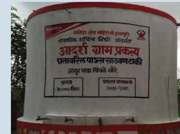
Rainwater tank, Awalkhed, Igatpuri, Nashik
