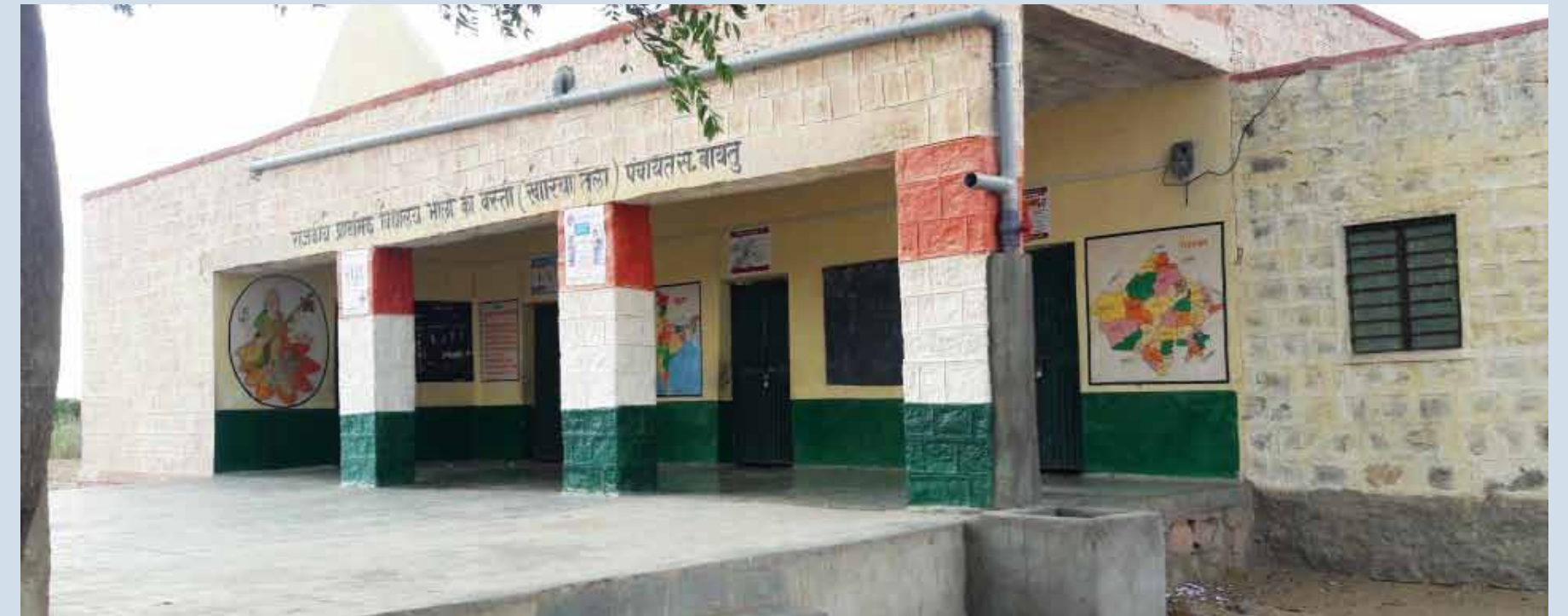
School Roof top RWH in Khariyatala, Barmer
