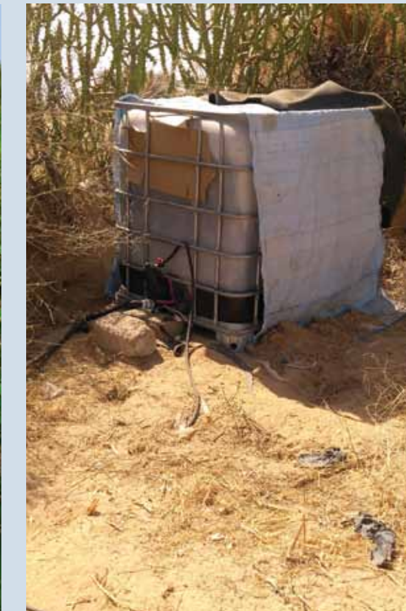
Gravity based drip, Bandra Talar, Barmer, Rajasthan
