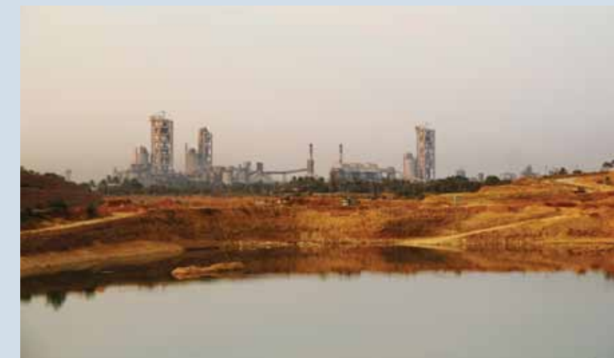
Recharging of mined out pits, Vadnagar, Kodinar Taluka, Gir Somnath District, Gujarat
