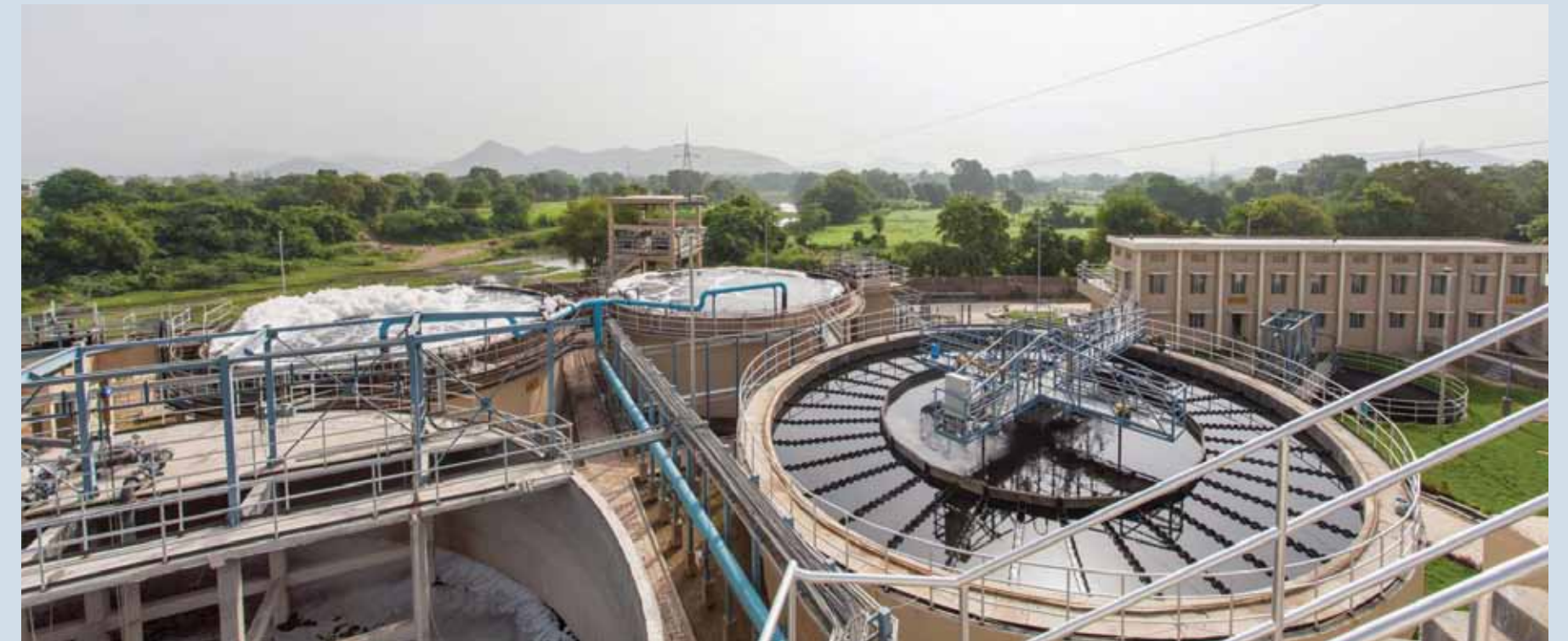
Sewage Treatment Plant using MBBR technology
