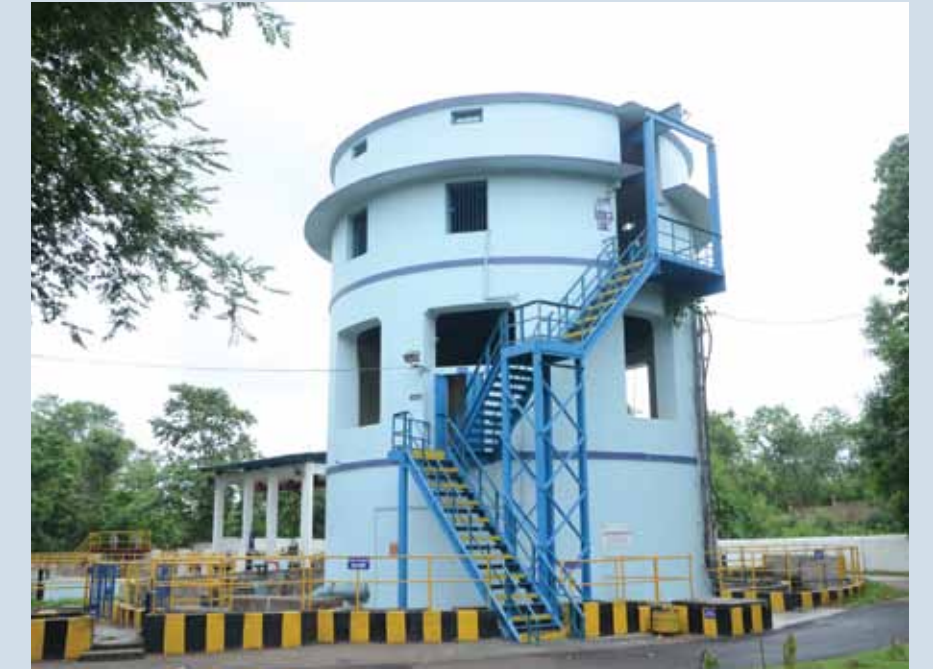
Sewage pumping station
