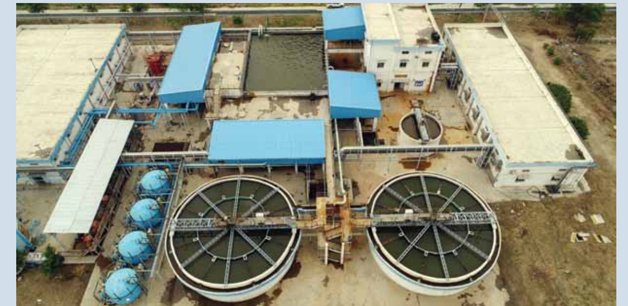
Water Treatment System
