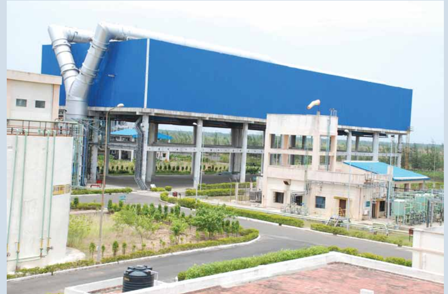
Air-cooled condensers
