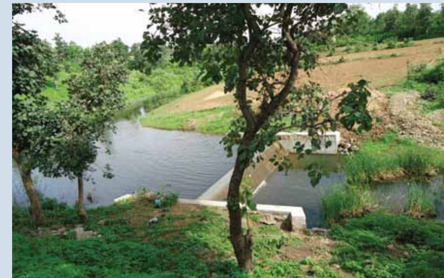
Check dam, Muripur
