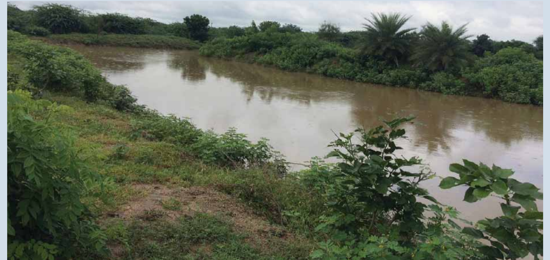
Earthen check dam, Ghanapur, Patancheru
