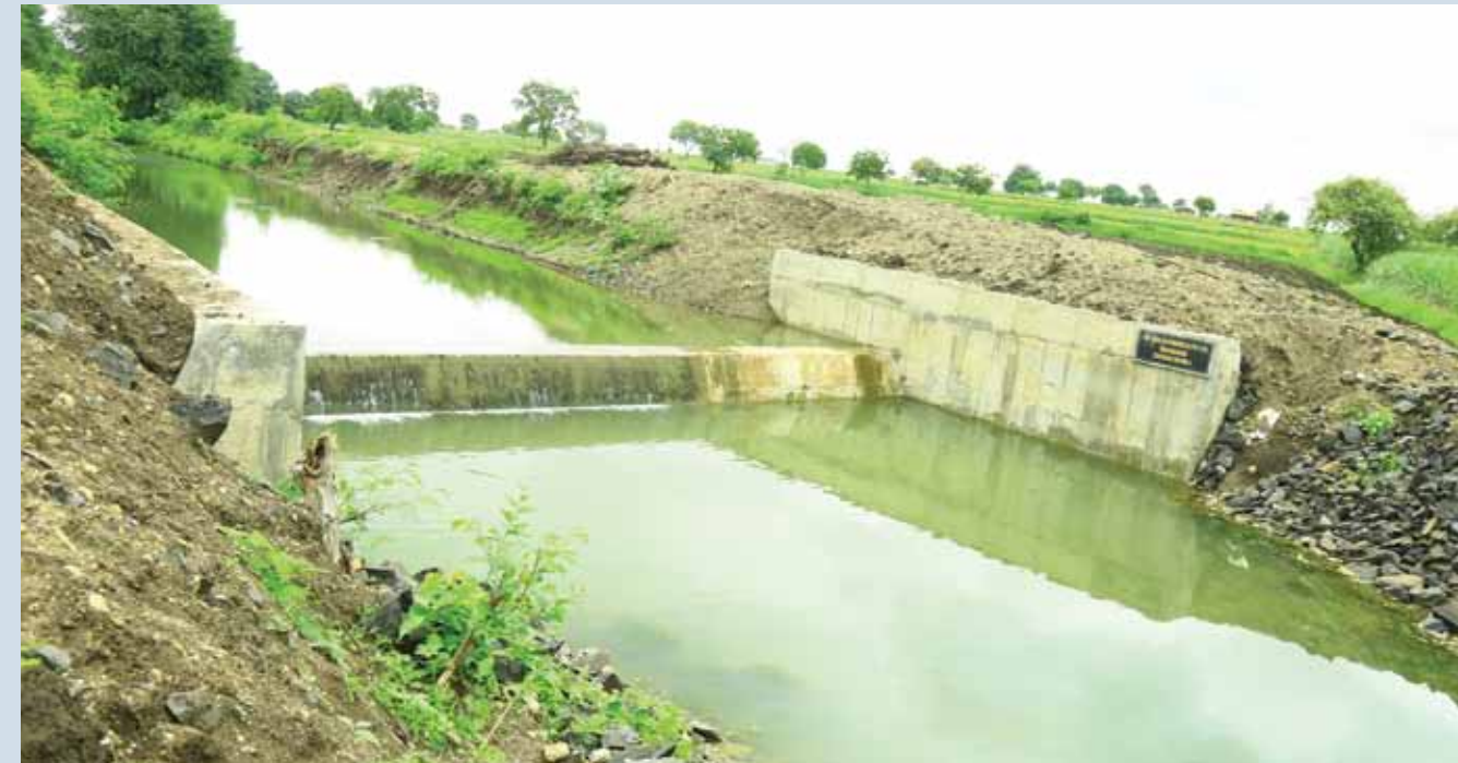
Construction of Cement Bahndhara and desilting of stream, Latur
