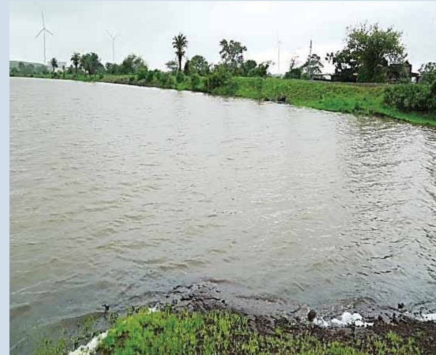
Rejuvenation of percolation tank, Chandrapur
