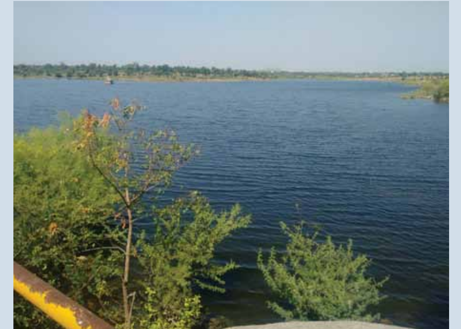
After: Ganga Sagar dam (Percolation tank) Dhamari Site
