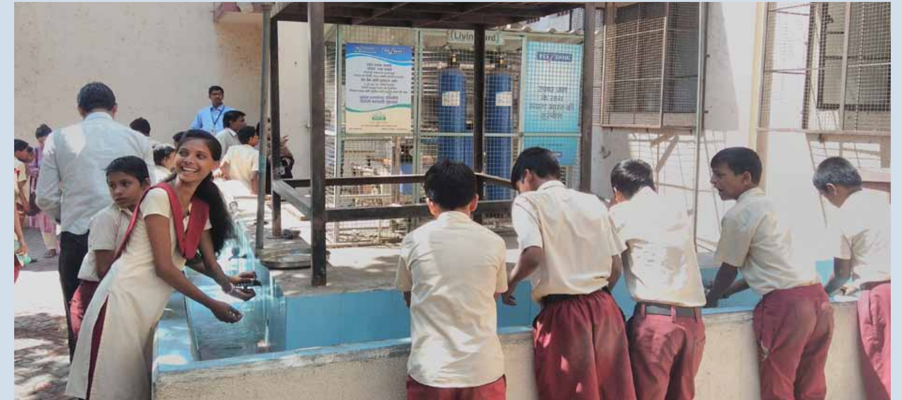
Drinking water system installed at Hamaal Panchayat Kashkari School, Pune
