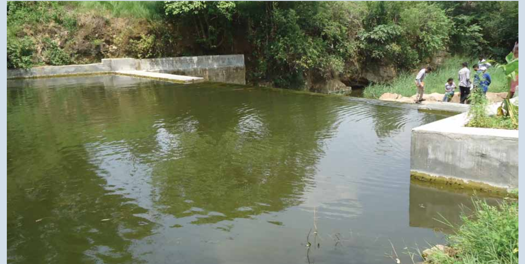
Check dam with Lift Irrigation
