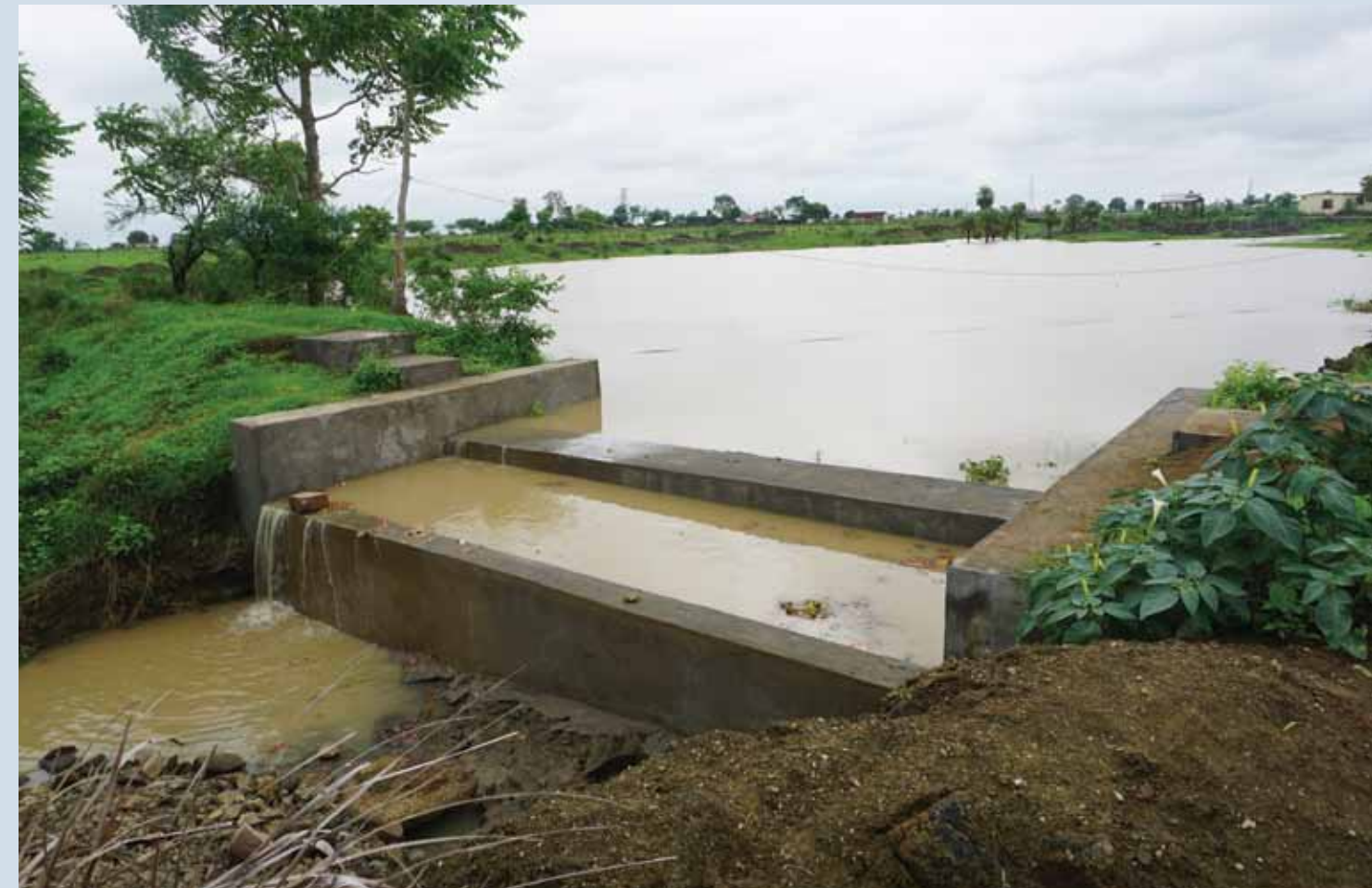
Revival of old village water tank, Jhagariakhurd, Bhopal
