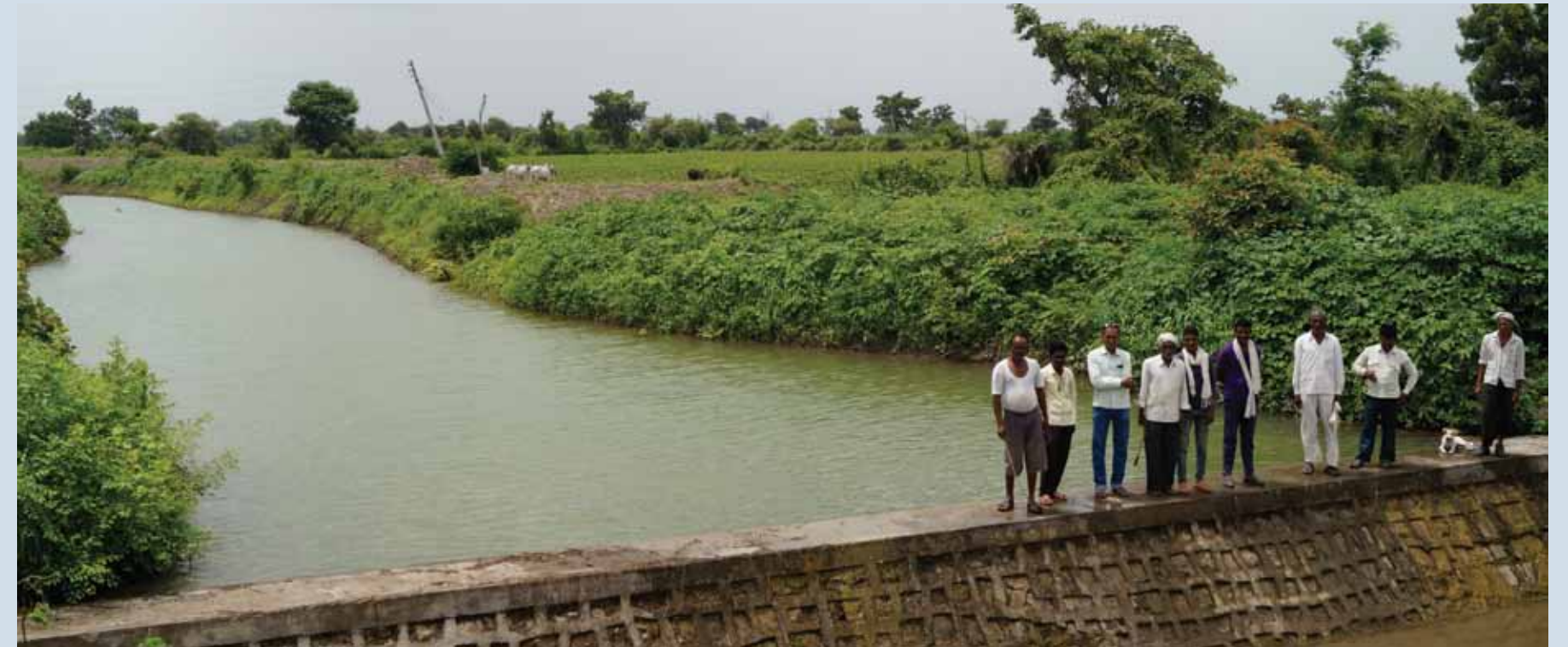
Check dam made functional at village Kawatha on Yashoda river, Wardha, Maharashtra
