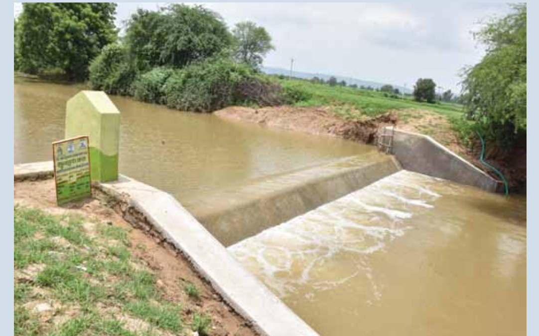
Check dam, Shrinagar, Bundi District
