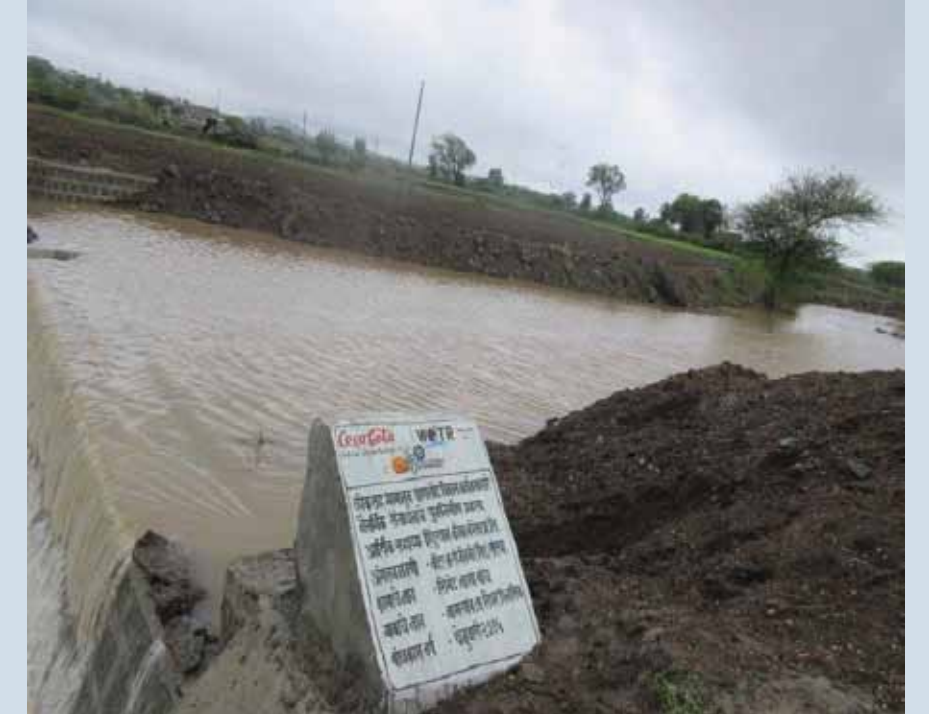
Construction of check dam, Jamgaon
