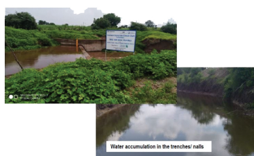
Check dams constructed at good water accumulation zones seen to be accumulating water
