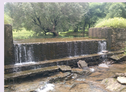
Checkdam at Kunda Village (Evaluation of Existing structures)
