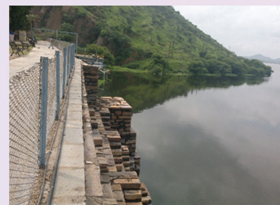
Pumphouse at Picchola Lake (Evaluation of existing drinking water schemes)
